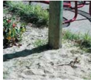
When a footing is below grade, staffers cannot perform a proper inspection. Landscaping in the image at left and sand in the image at right hide the footings from the inspector.
