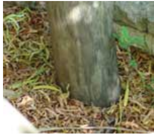
When a footing is below grade, staffers cannot perform a proper inspection. Landscaping in the image at left and sand in the image at right hide the footings from the inspector.
